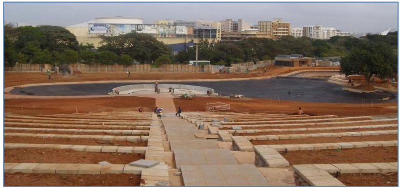
Placement of Sealmac® & coating with Waterbloc bitumen
