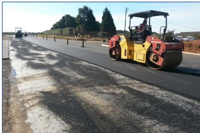
Gravel spread over Sealmac ® under a 50mm asphalt layer
