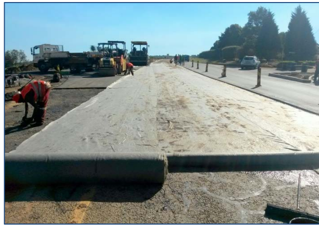
Sealmac ® was laid over bitumen on milled surface
