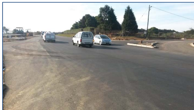
The repaired road surface
